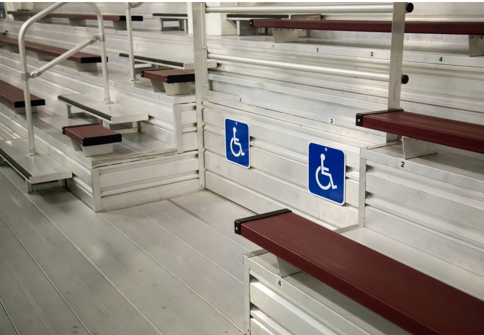
Image Description: empty bleachers with an open space in the middle for a mobility device.
