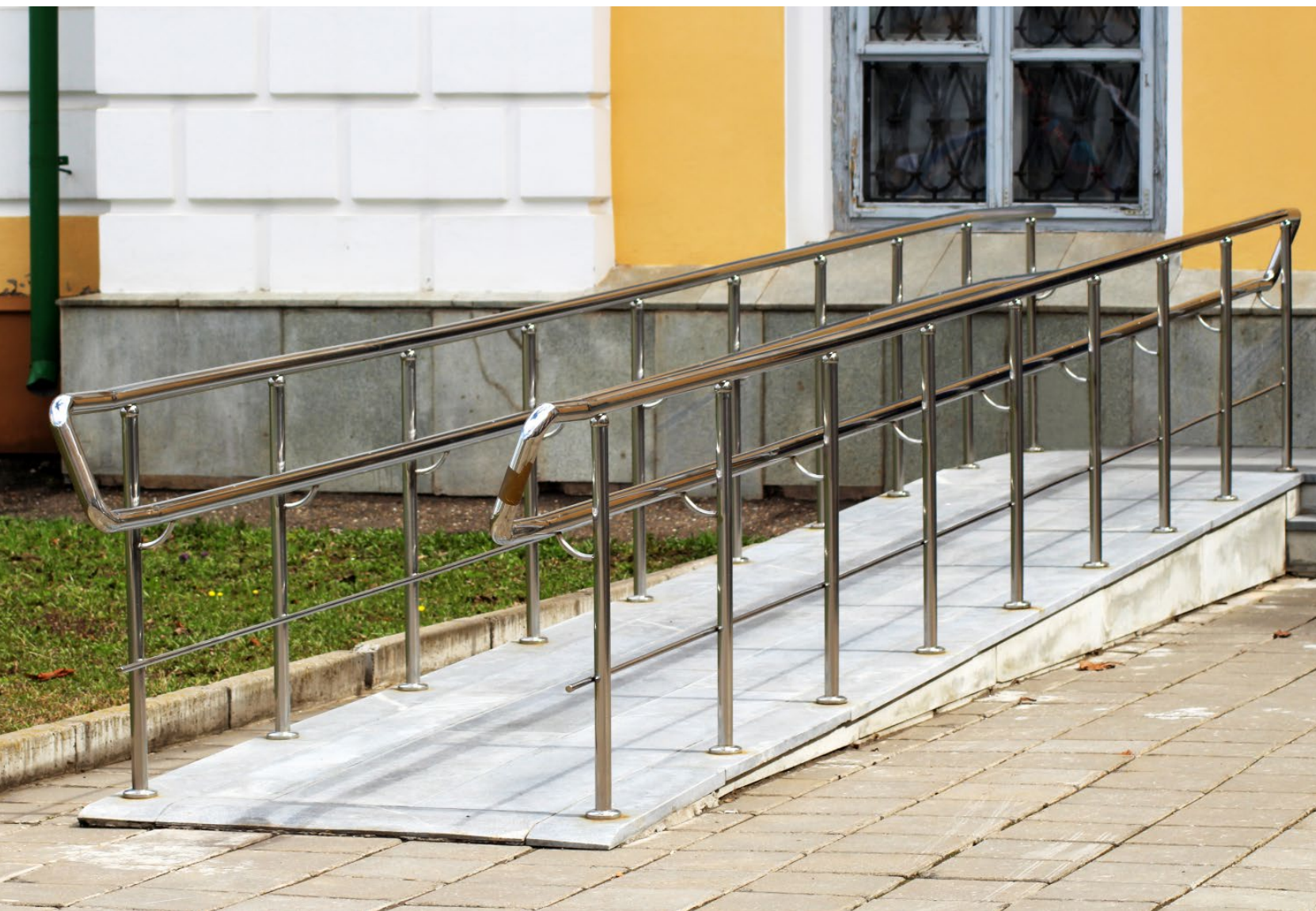
Image Description: An entrance to a building with two stairs as access. A concrete ramp has been built over the stairs with secured, steel handrails.
