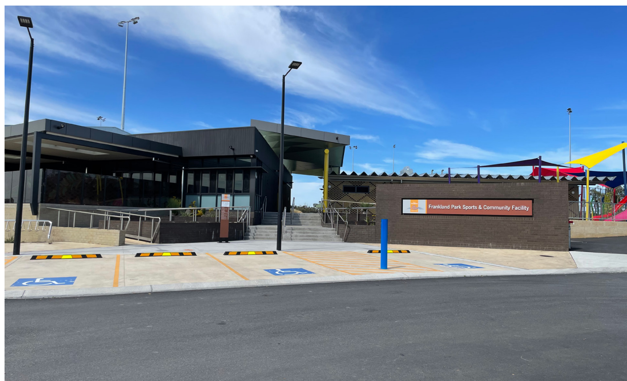
Frankland Park Sports & Community Facility, Hammond Park, WA
