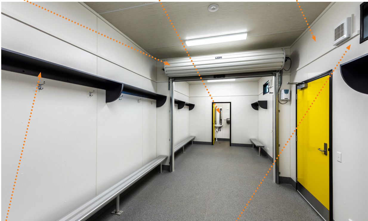
Overhead storage and coat hooks
